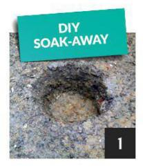
Dig a new hole at the bottom of the main hole about 2ft (24") in diameter and about 2ft (24") in depth.
