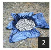
Line the hole with a permeable weed membrane (available at most DIY stores) and fill with scalpings, shingle or just crushed hardcore. The membrane will stop the hole silting up and allow water to collect and drain properly.
