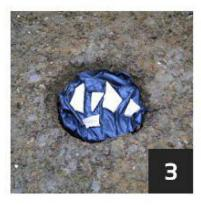
Finally wrap the membrane over the top of the hardcore/ shingle/scalpings and lay some slabs on top to seal the top. You now have a very effective soak-away.
