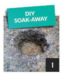
Dig a new hole at the bottom of the main hole about 2ft in diameter and about 2ft in depth.
