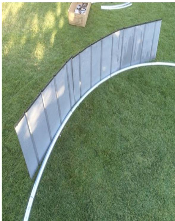
**Step C: Join the upper frame segments to the wall panels.**
